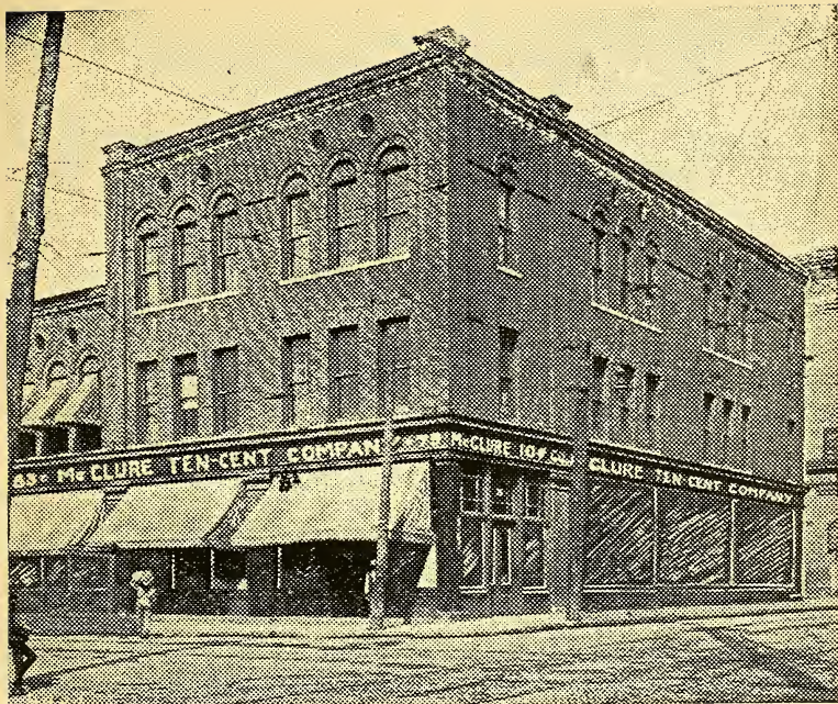
General Offices and Retail Store of McClure Ten Cent Company, McClure Building, Mitchell and Forsyth Streets, Atlanta, Ga.
